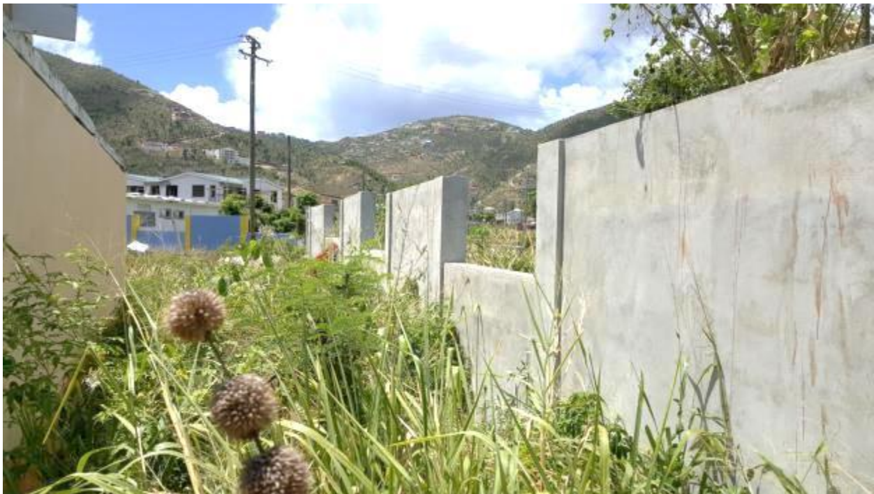
Photo 8: Area 2 (Unpainted Wall approaching Evans House)
