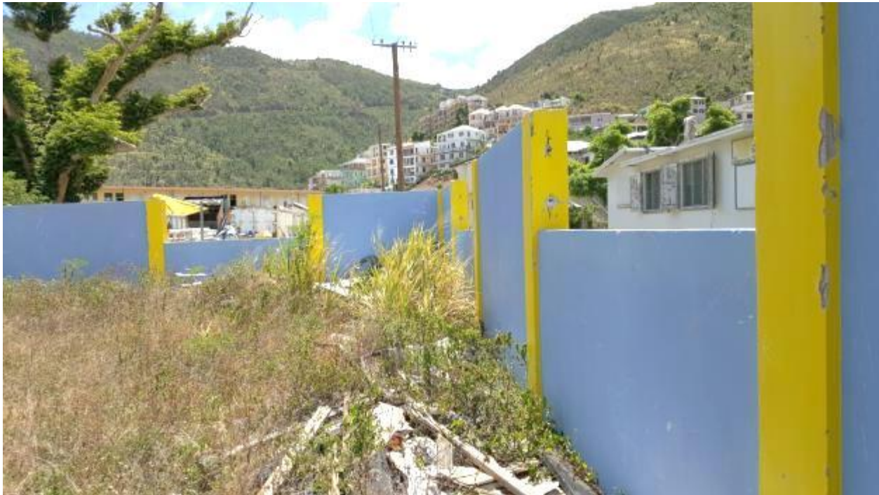
Photo 11: Area 3 (Finished Wall behind Evans House )
