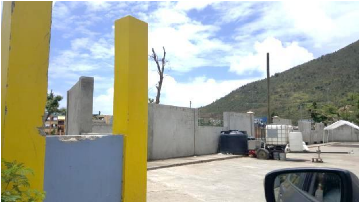
Photo 5: Area 1 (Bus Stop Modification to project)
