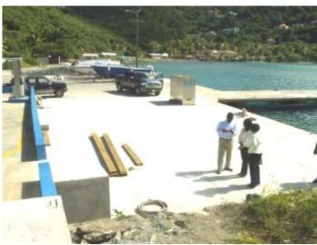
20. Phase II of the dock is deemed to be structurally sound and it is felt that it can potentially house a two story building and function as a port of entry. Presently, however the facilities are primarily used by pleasure boaters and fishermen.
